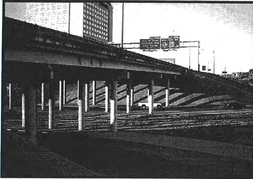
Figure 7: Interstate 35 Separating the Neighborhood from Downtown
