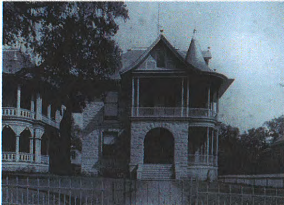
910 West 6 th Street, now demolished.
